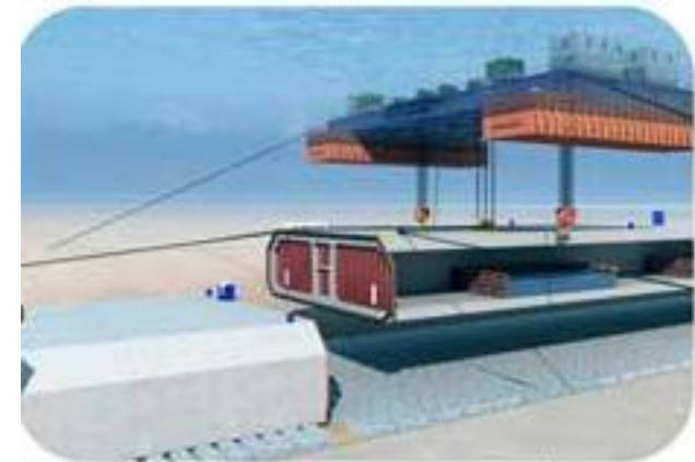
Tube installation
